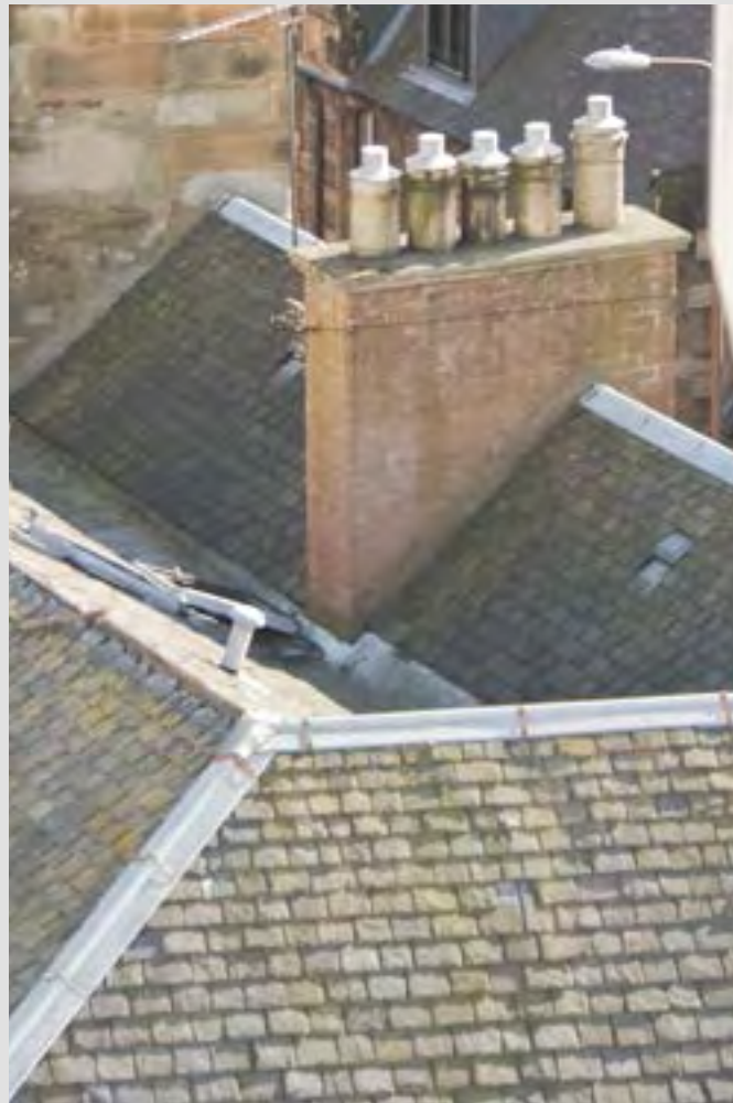
Traditional roofing materials (right) Slate, Lead and zinc are traditional roofing materials used in Edinburgh—seen here from the Museum of Scotland’s roof
