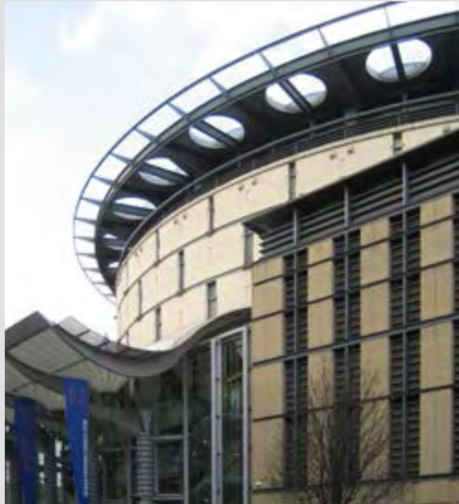
A mixture of cast stone & natural stone—Morrison St. Cast stone was used at high level on the drum shaped part of the building while natural stone was used at low level on the corners.
