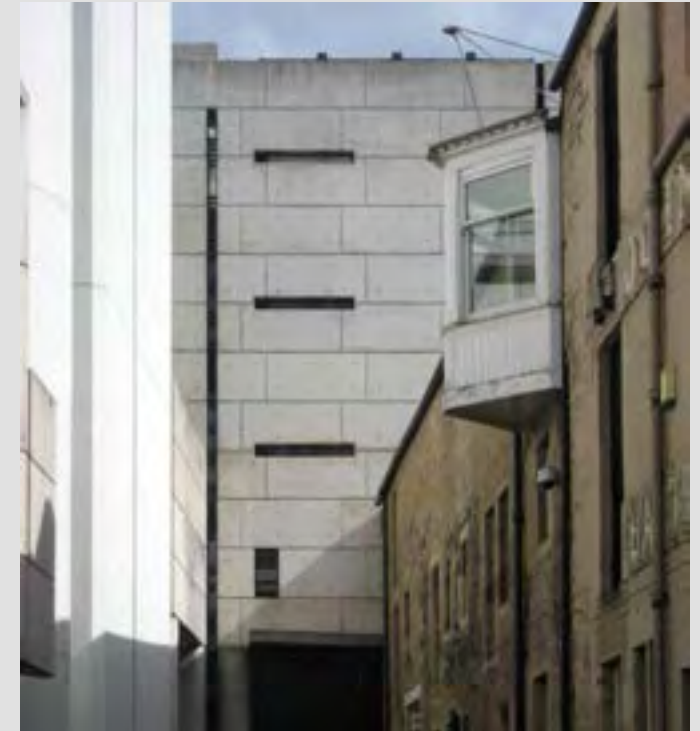
In-Situ Concrete—Museum of Scotland This concrete is used to sculptural effect on the museum building
