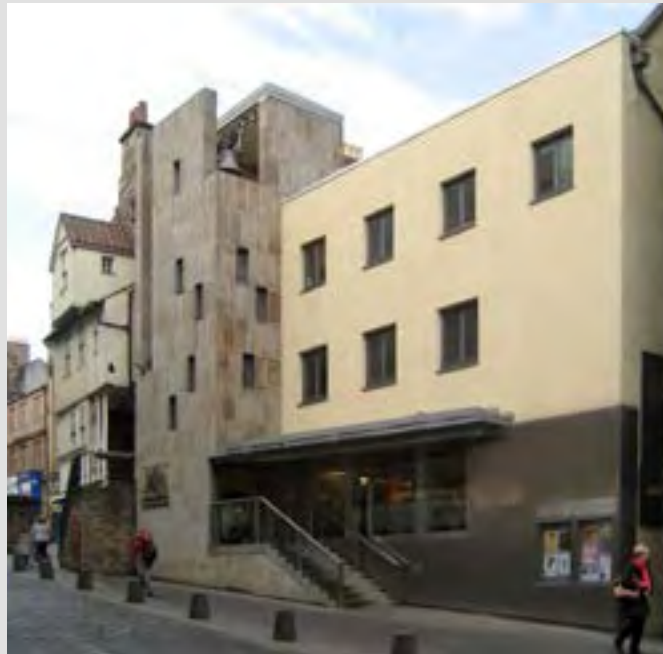
Integrating the new with the old—High Street
