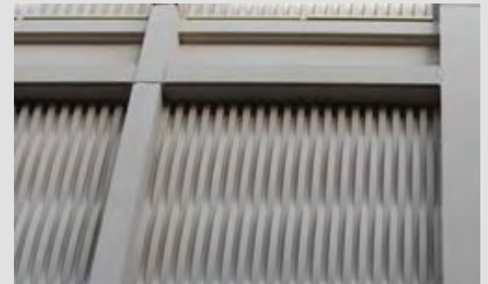
Textures created with concrete—Princes Street Concrete panels with textured surface treatment are used on this recent building on Princes Street.
