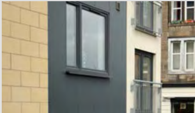
Too many materials? The cladding, blockwork and render and their detailing used at this development would not now meet the Council's expectations for appropriate quality.
