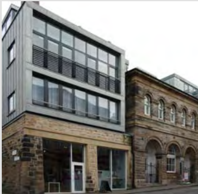
Using zinc to provide striking contrast—Infirmery St. The zinc cladding combined with the modern building form provides a positive contemporary contrast to the historic former Infirmery Street Baths building.
